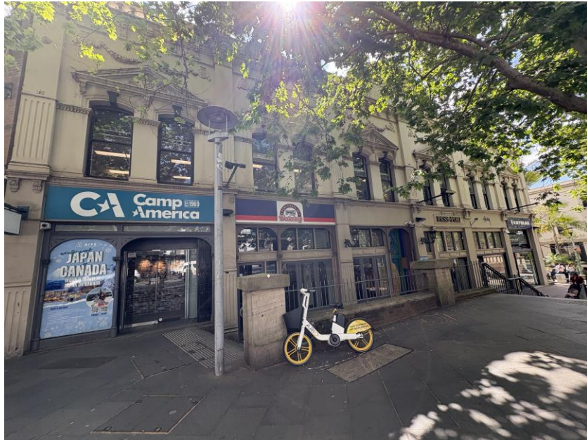
Figure 1: 10-14 Oxford Square, Darlinghurst, viewed from the south
